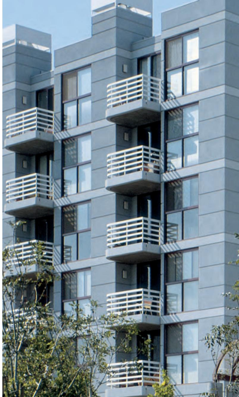
Exterior continuous insulation (CI), as well as an air barrier, are the most effective ways to [meet both Federal and California energy code requirements](#). Exterior Insulation and Finish Systems (EIFS) are a proven methodology that integrates these elements into a durable, design-flexible, cost-effective, single source solution that fully meets and exceeds the new codes.
