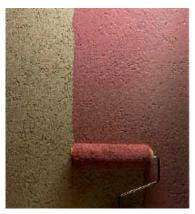
the surface shall be thoroughly washed with muriatic acid and flushed to remove residual acid. All projections shall be removed and small voids filled with Primus®, Primus DM, or Genesis® mixture.
